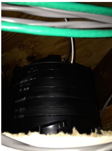
A side view of one of the installed Beale Street Speakers shows how massive the Sonic Vortex back box is.
