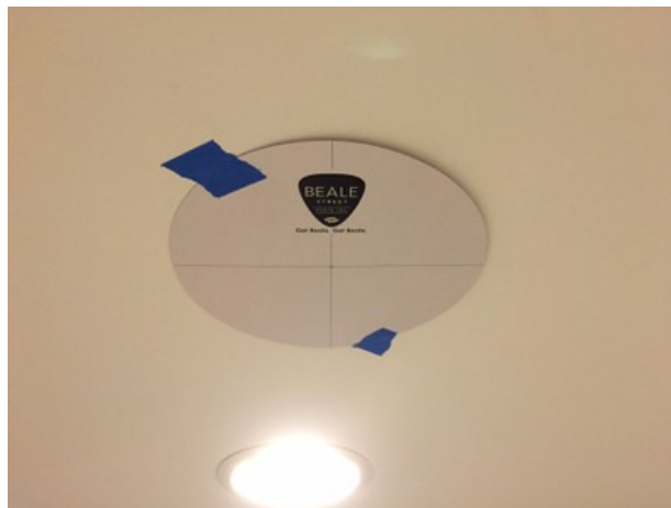
Beale Street's template make it easy to trace the proper speaker cut out diameter.
