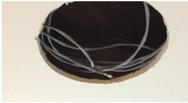
The Blue Jeans Cabling was run and clearly labeled on either end for easy matching later on.
